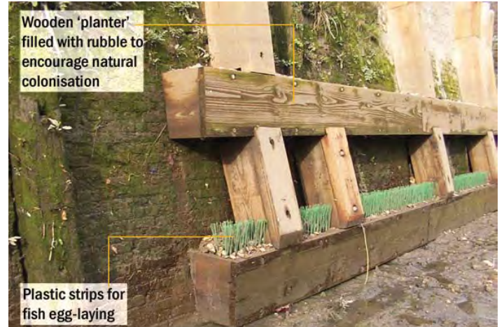
DEPTFORD CREEK, LONDON: TIMBERING TO RIVER WALL
