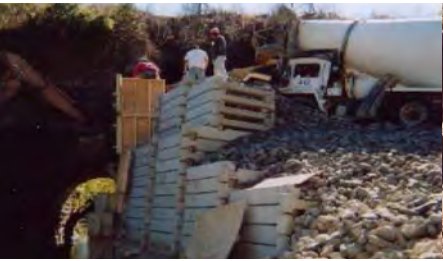
CONCRETE CRIBBING INSTALLATION
