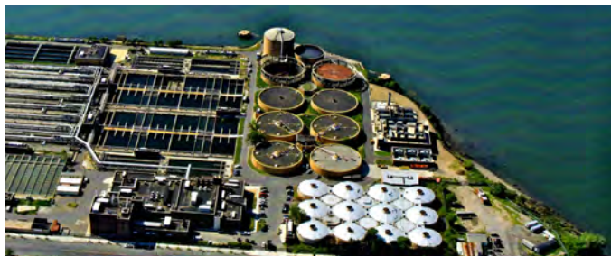
Hunts Point Waste Water Treatment Plant
