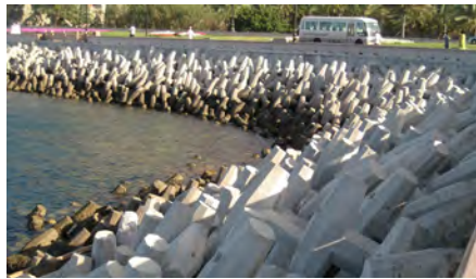
CONCRETE JACK INSTALLATION-UAE
