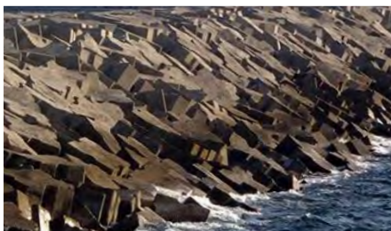
ECONCRETE SHORELINE STABILIZATION
