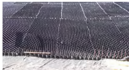
STEEP SLOPE INSTALLATION
