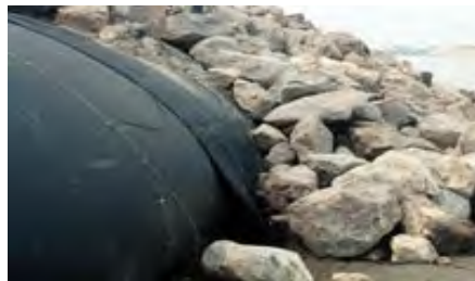
COVERED WITH RIPRAP
