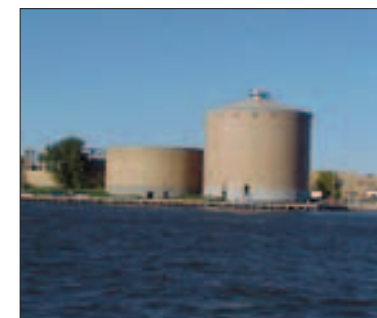
Water Pollution Control Plant
