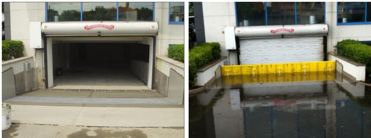
Figure 8. Example of Dry-Floodproofing
